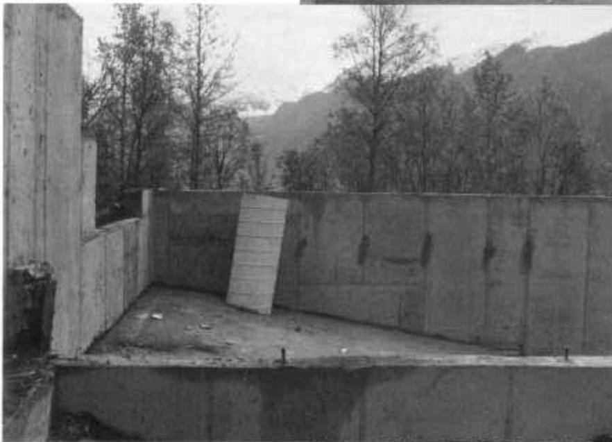
Upper end of greenhouse pit before back-filling. The 16"-diameter duct is connected to the air return plenum below the slab.
