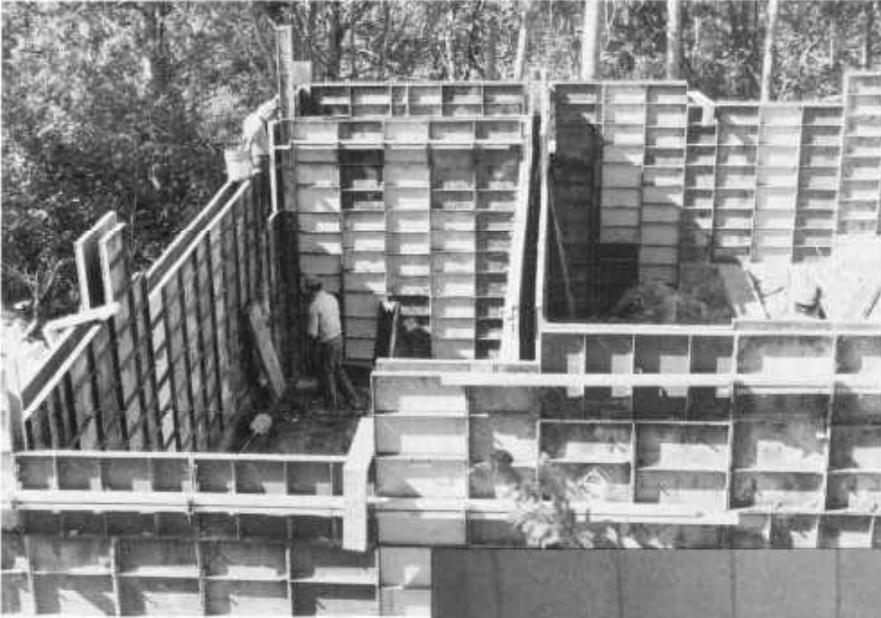
The concrete formwork in place. The greenhouse pit is to the left (with the man inside it) and the cistern beyond it (12 ft deep).
