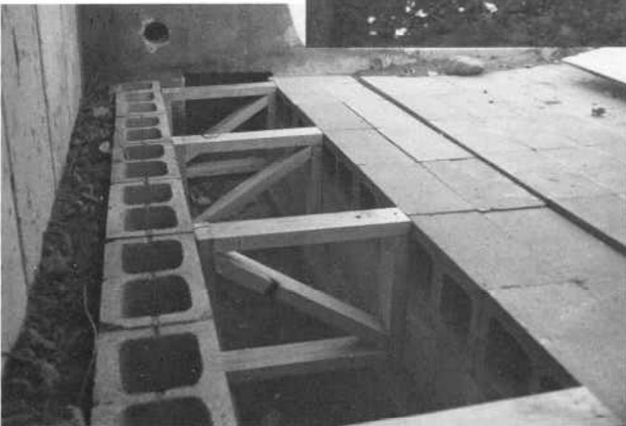
View of supply plenum and duct opening to the mechanical room beyond. Note 4" drain pipe penetration.
